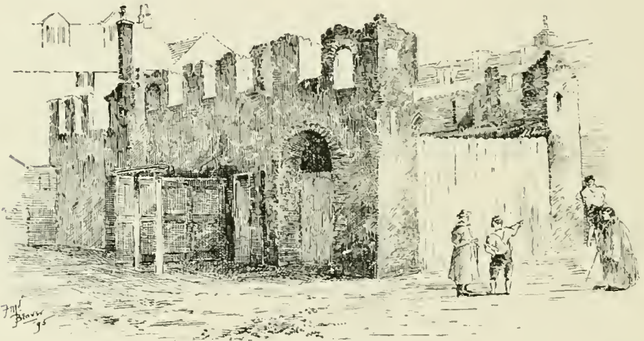
RUINS OF THE THEATRE IN BEAR YARD.
